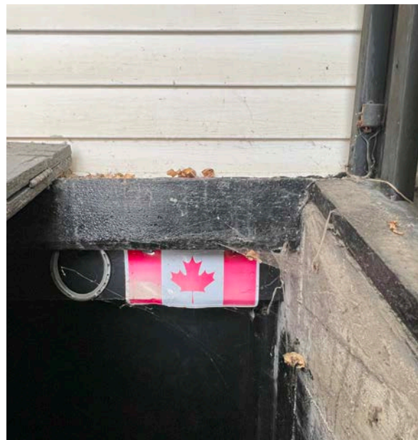
Timber lintel over the basement door at the rear (west) elevation provides evidence of an older structure (ERA, 2025).
