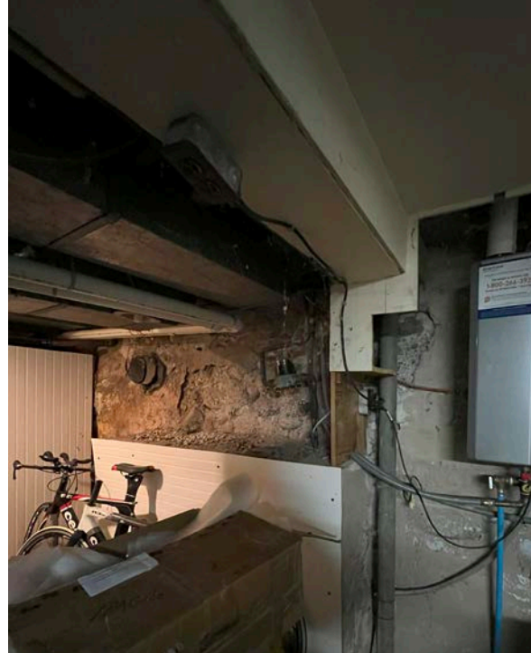
Stone foundation wall underneath cement parking (ERA, 2025).
