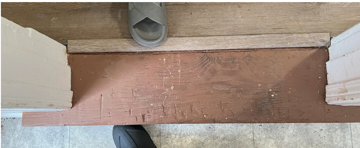
Entrance to the smaller unit at 12 Spruce Street; door sill, jamb, baseboard, and baseboard plinth block provide evidence of an older structure (ERA, 2025).
