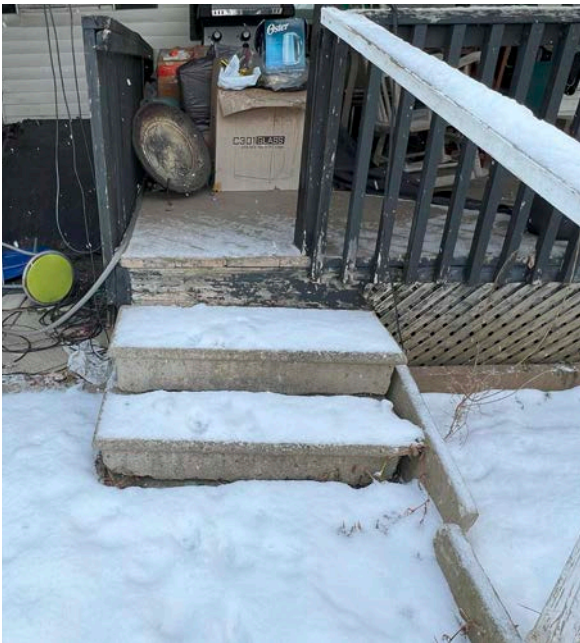
Painted wood on the rear porch in fair to poor condition (ERA, 2025).
