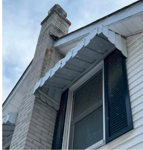
Modern vinyl windows and metal awnings and shutters at the north (side) elevation in fair condition. Modern brick chimney in fair condition with minor deterioration towards the top (ERA, 2025).
