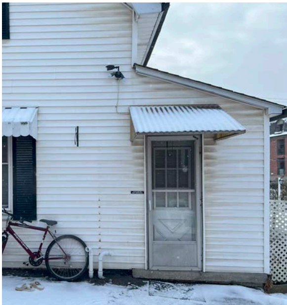
Vinyl siding at the north (side) elevation in fair condition, with some soiling and organic growth visible (ERA, 2025).
