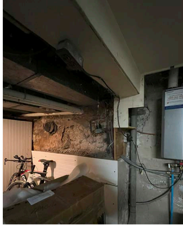
Stone foundation wall underneath cement parking (ERA, 2025).
