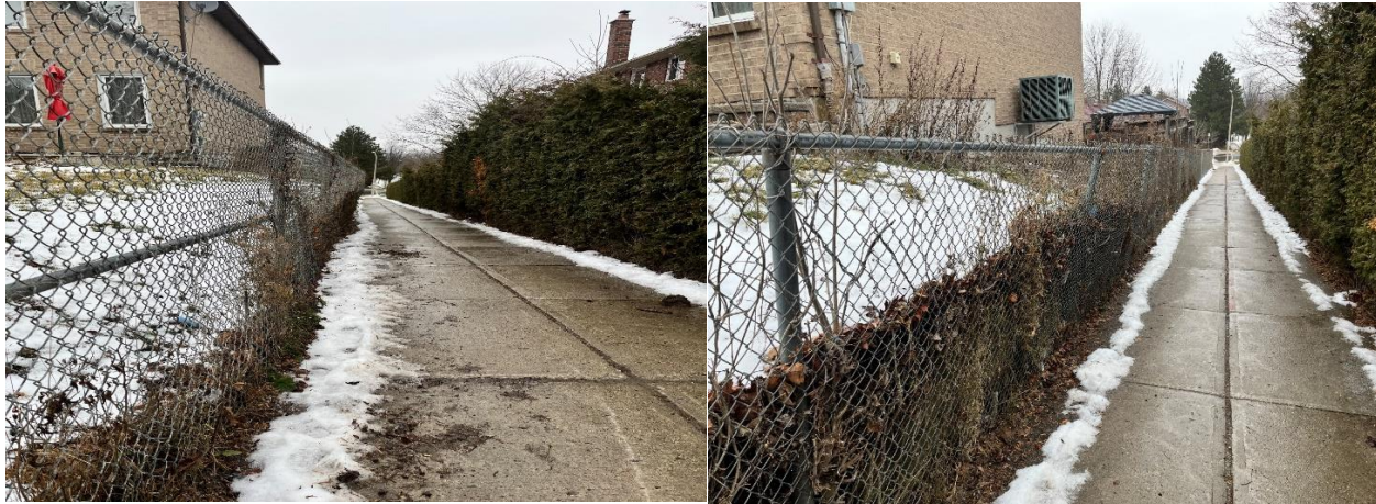
Figure 3 – Images of the failing retaining wall with the chain-link fence leaning into the walkway:
