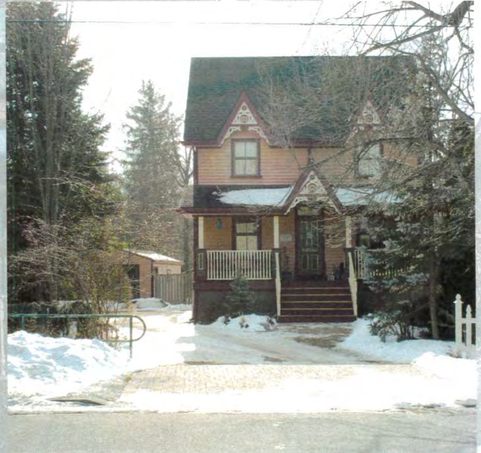
After: Higher roof, new porch, new bargeboard, new foundation, new windows and doors
