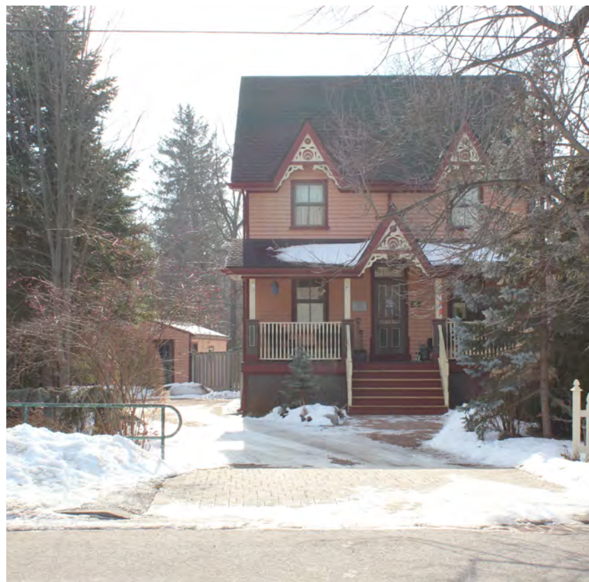
After: Higher roof, new porch, new bargeboard, new foundation, new windows and doors
