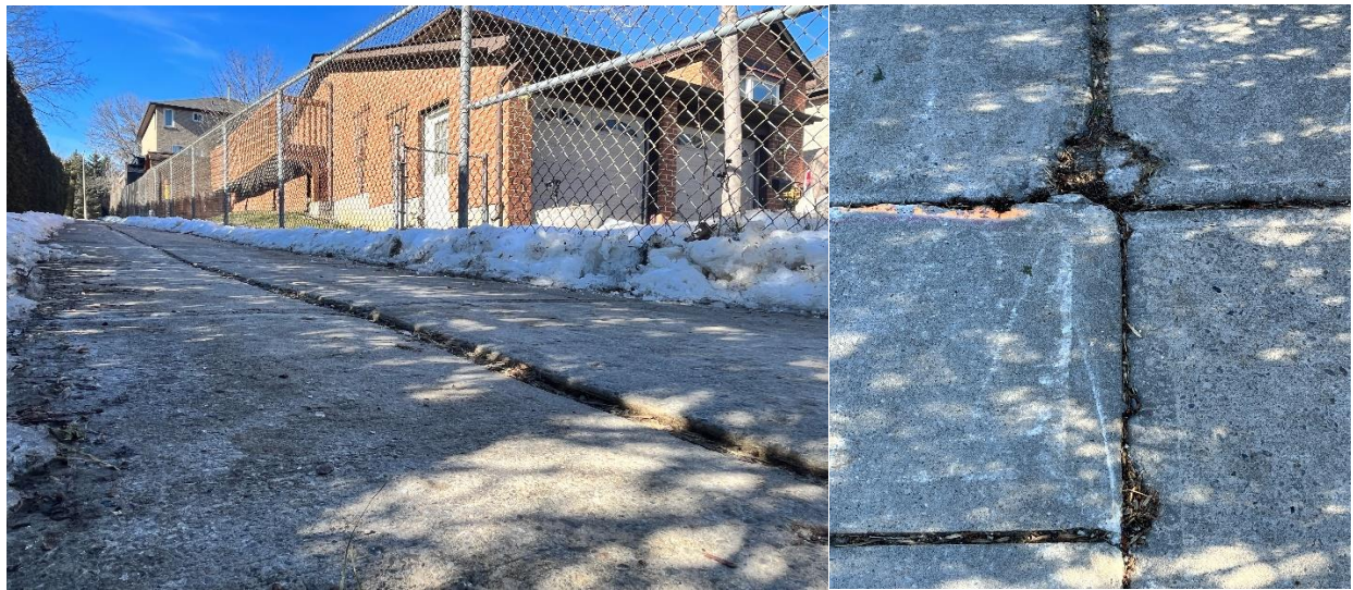
Figure 6 – Longitudinal joint deflections and uneven walking surface:
