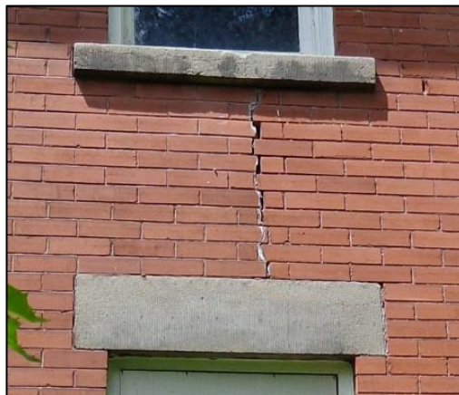
Figure No. 5.7 Masonry cracks – south wall (left and west wall (right
