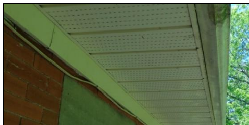
Figure 5.12 Existing soffits, frieze, fascia and eaves troughing (left), shingles (right).
