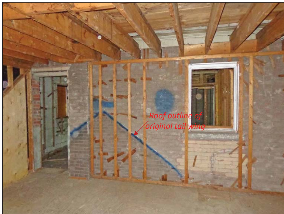
17. Room 11 – East wall showing roof line of original addition
