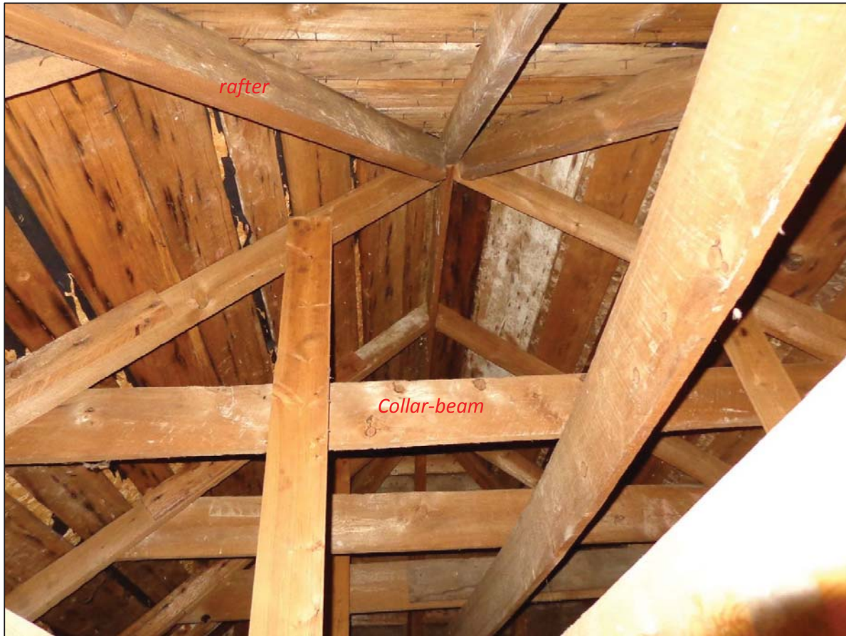
6. Attic – Roof framing – view to the north side
